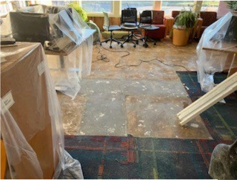
Carpet ripped out from extensive water damage.
