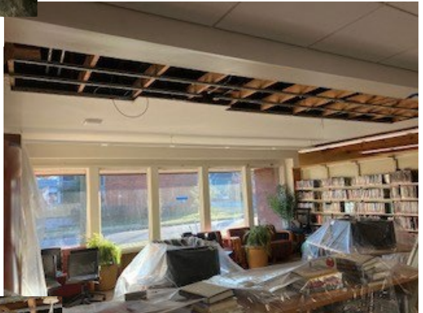
Damaged ceilings and covering computers until they can be removed.
