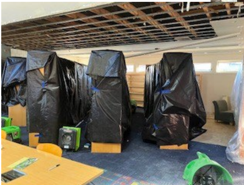
Extensive ceiling damage. Covered existing shelving.
