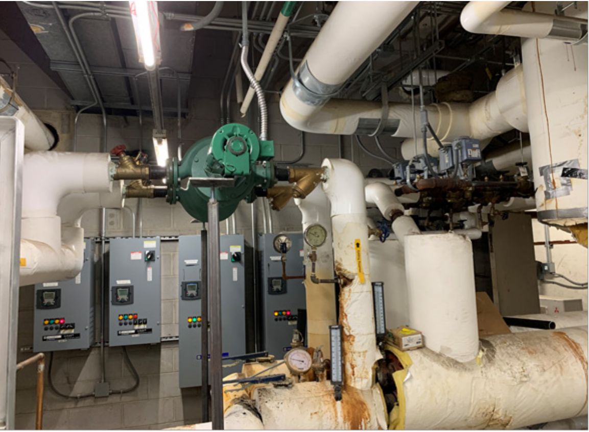
Figure M3 Existing Steam - Hot water converter installed in 1970s
