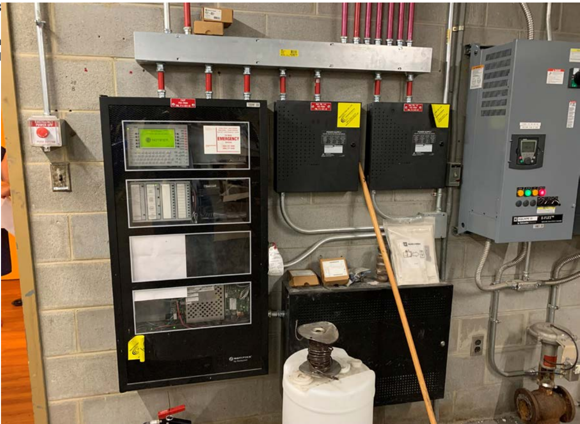
Figure E3 Existing Fire Alarm Control Panel
