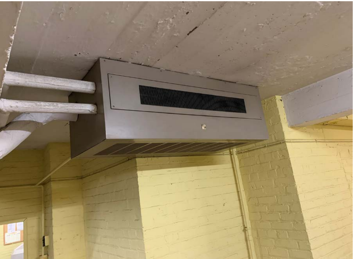
Figure M7 Existing Induction Units serving part of Dooley Building
