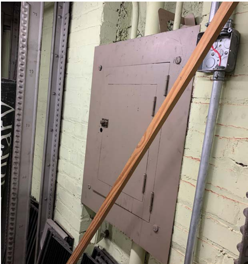
Figure E2 Typical Existing Panelboard
