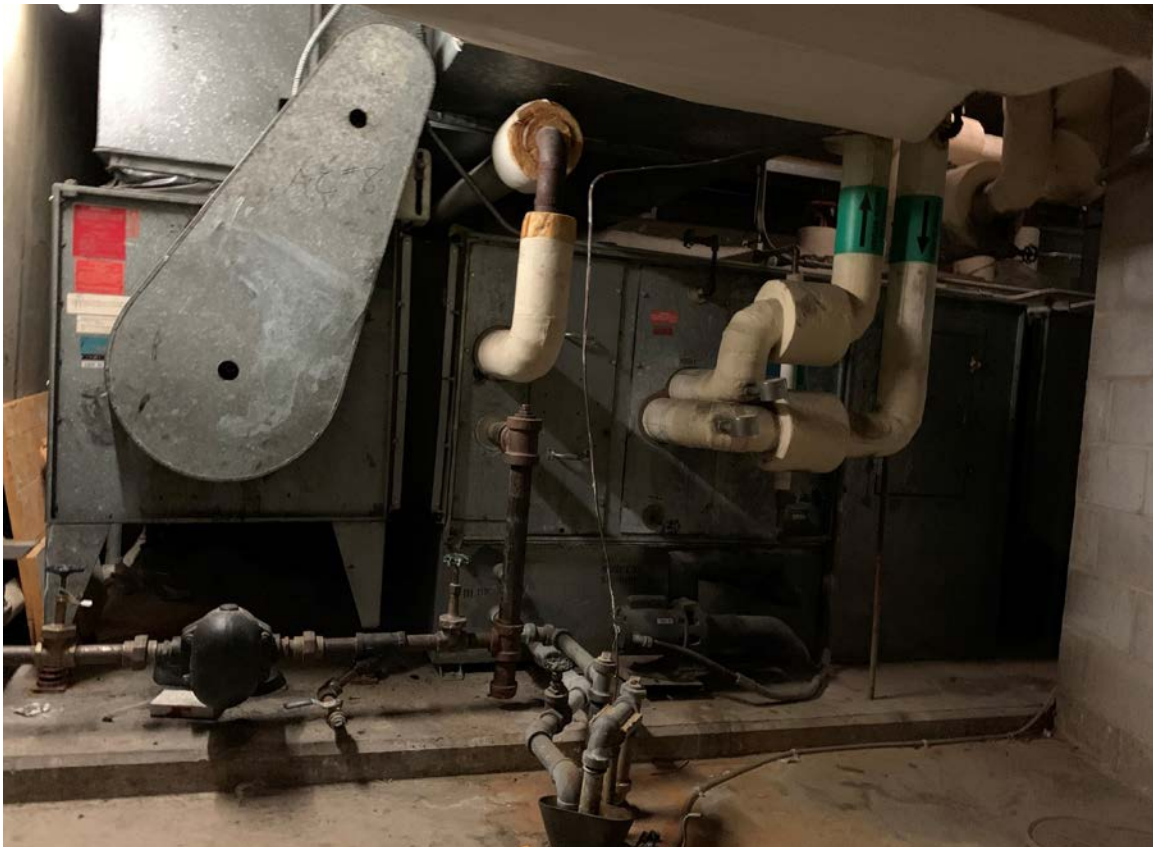
Figure M5 Existing Multi-zone Air Handling Unit installed in 1970s
