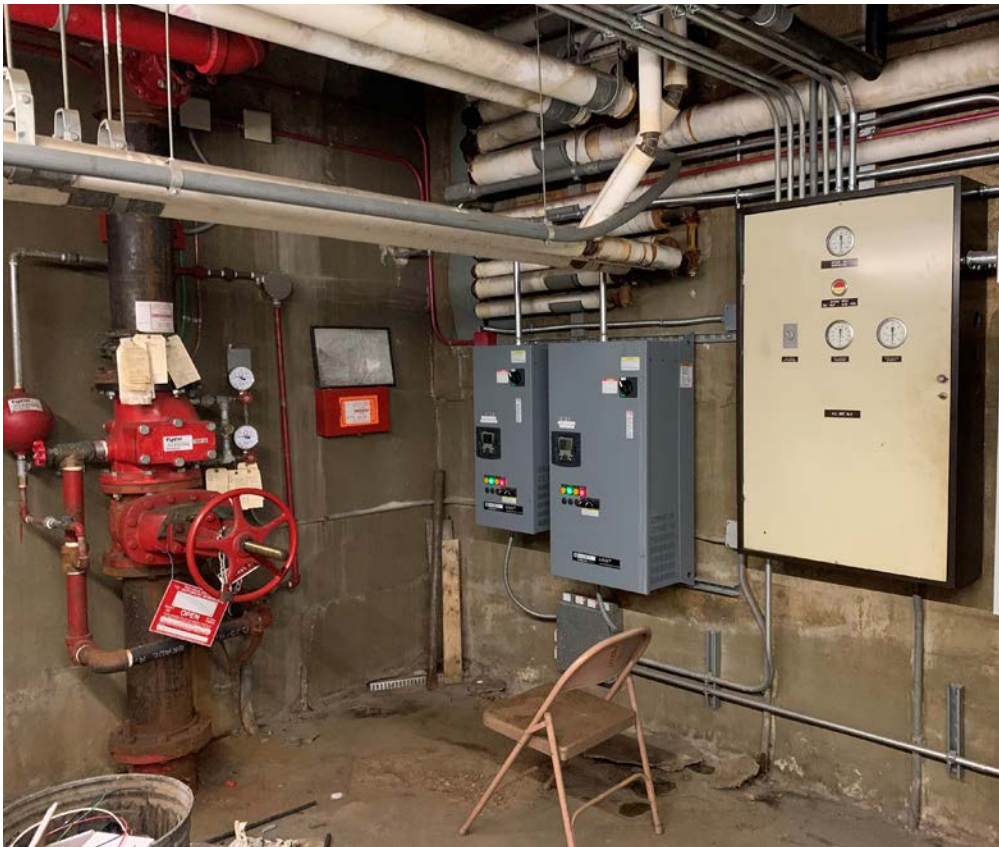
Figure P2 Existing Dry-pipe Sprinkler Valve
