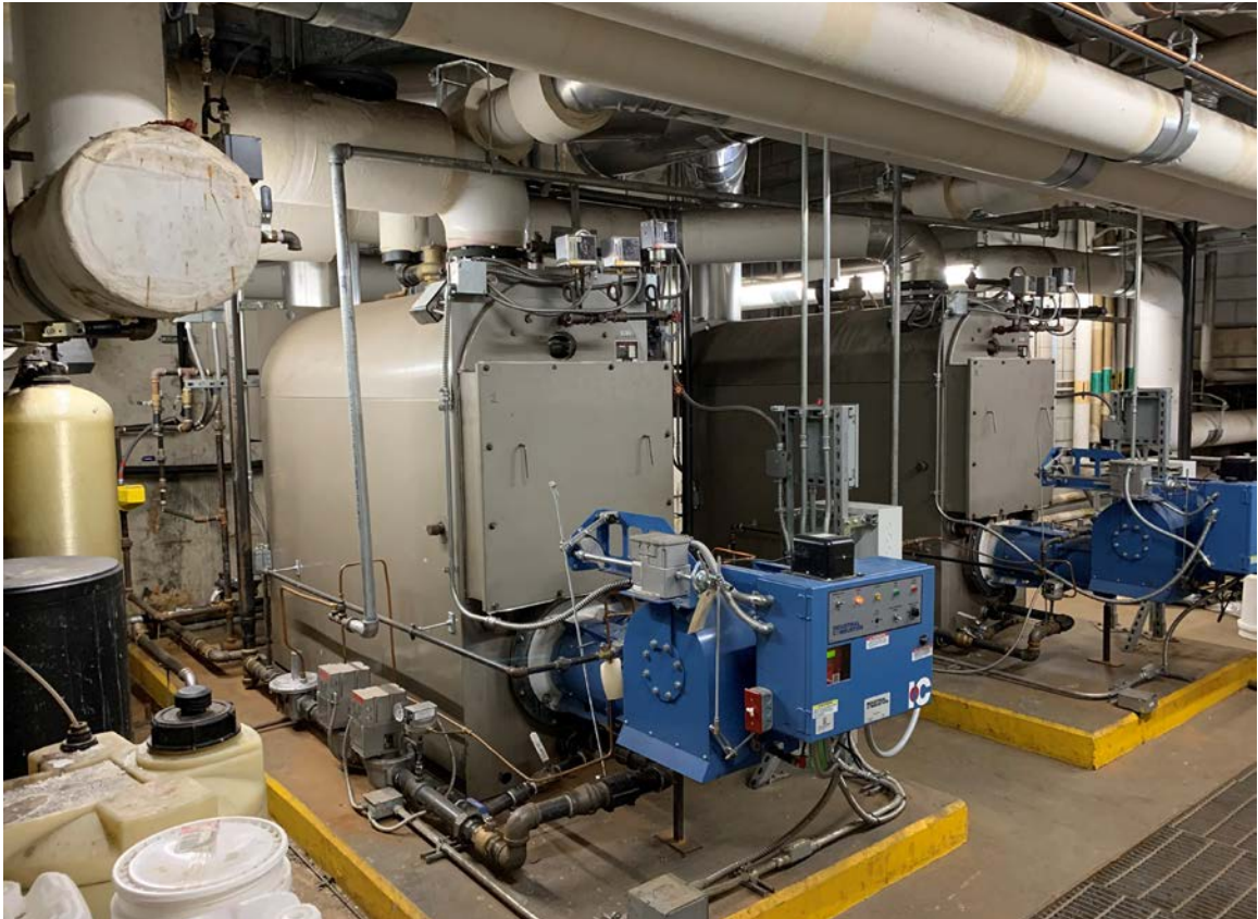
Figure M2 Existing Steam Boilers
