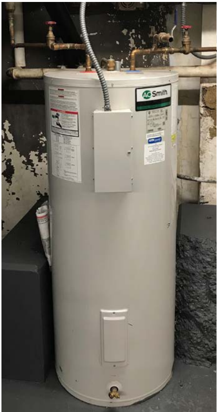
Figure P1 Existing 80-gallon Electric Water Heater
