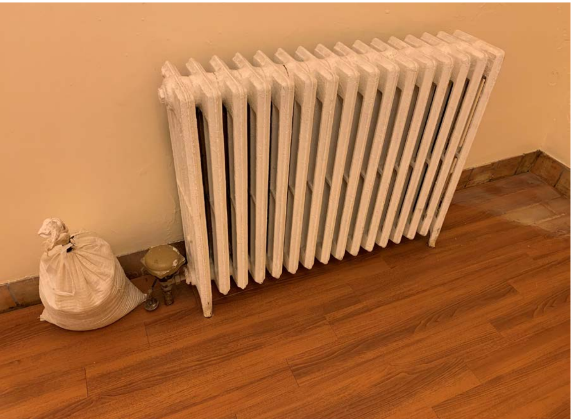
Figure M8 Existing Hot Water / Steam Radiator
