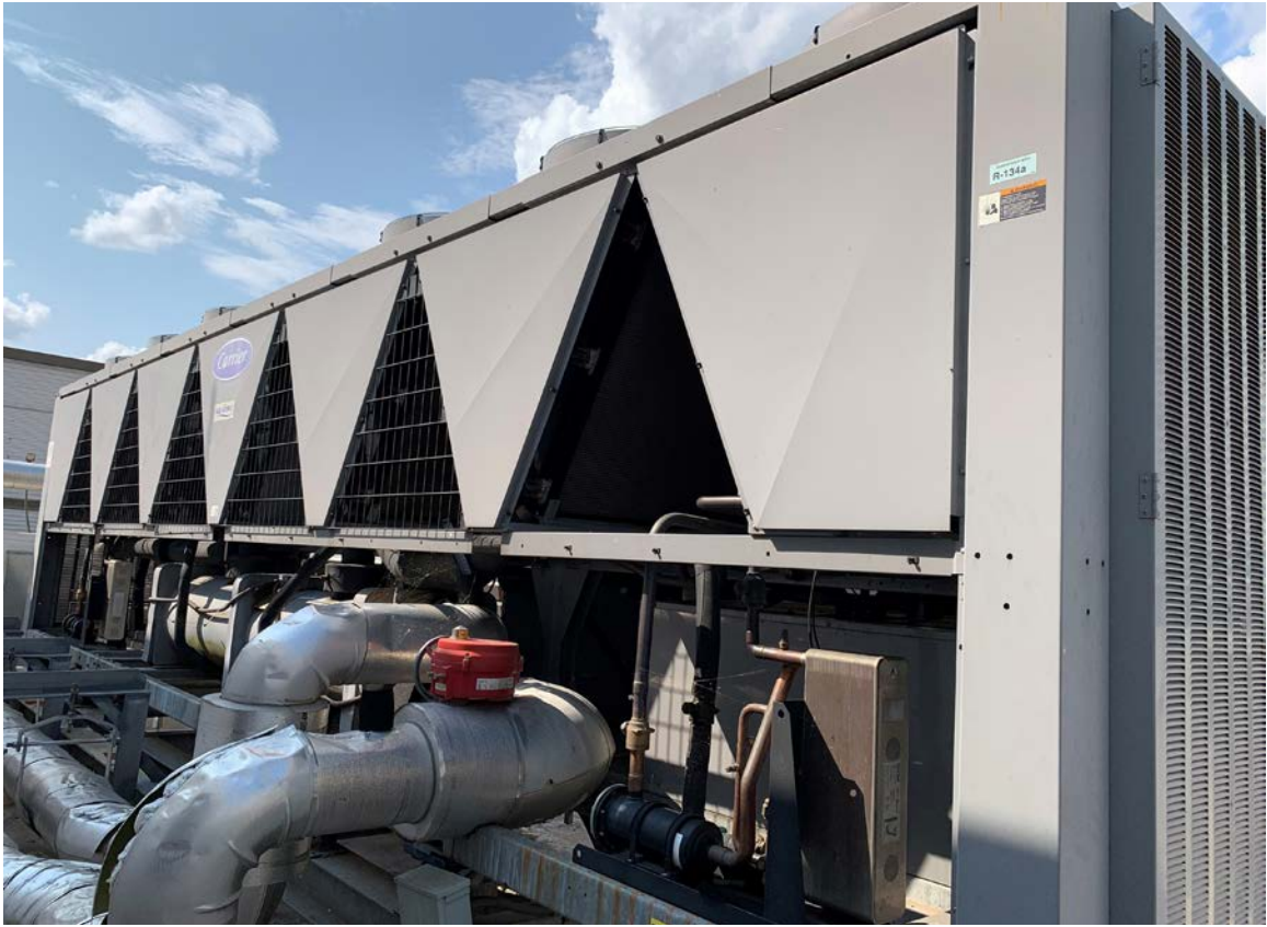
Figure M1 Existing Air-cooled Chiller
